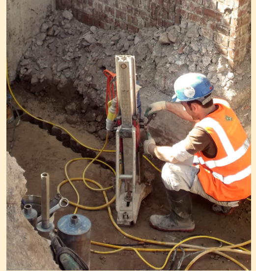
Diamond drilling for chapel stabilisation works
