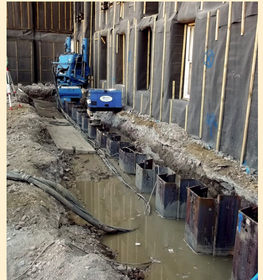
Stabilisation works on Nassau Street
